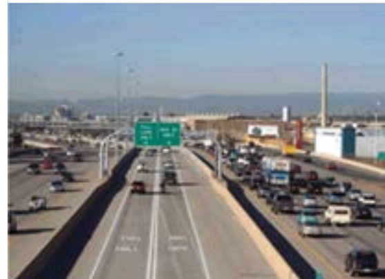
Concrete Safety Barrier
